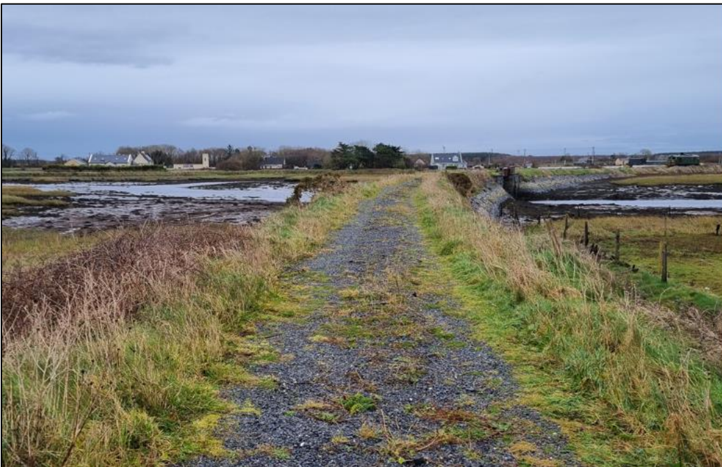
Plate 4.2 Ch. 7+750 looking east over Moyasta Bridge.
