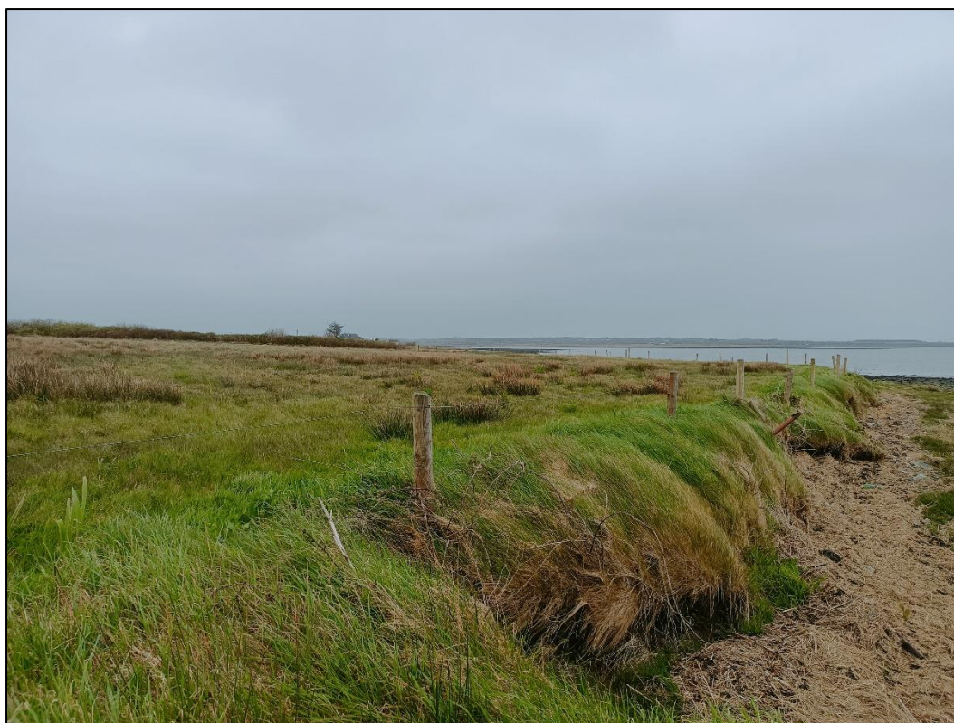
Plate 2.1 View at Ch. 6+300 looking east.
