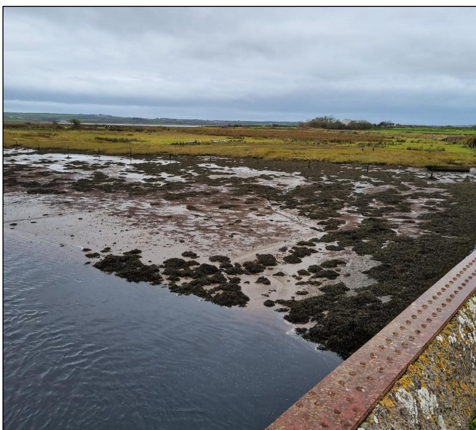
Plate 4.4 View off Moyasta Bridge looking west.
