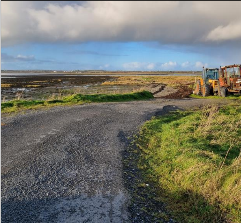
Plate 6.1 Existing roadway at Ch. 9+800 where greenway will be routed. Tractors on the right-hand side of the photo are used to access oyster trestles in the Bay.
