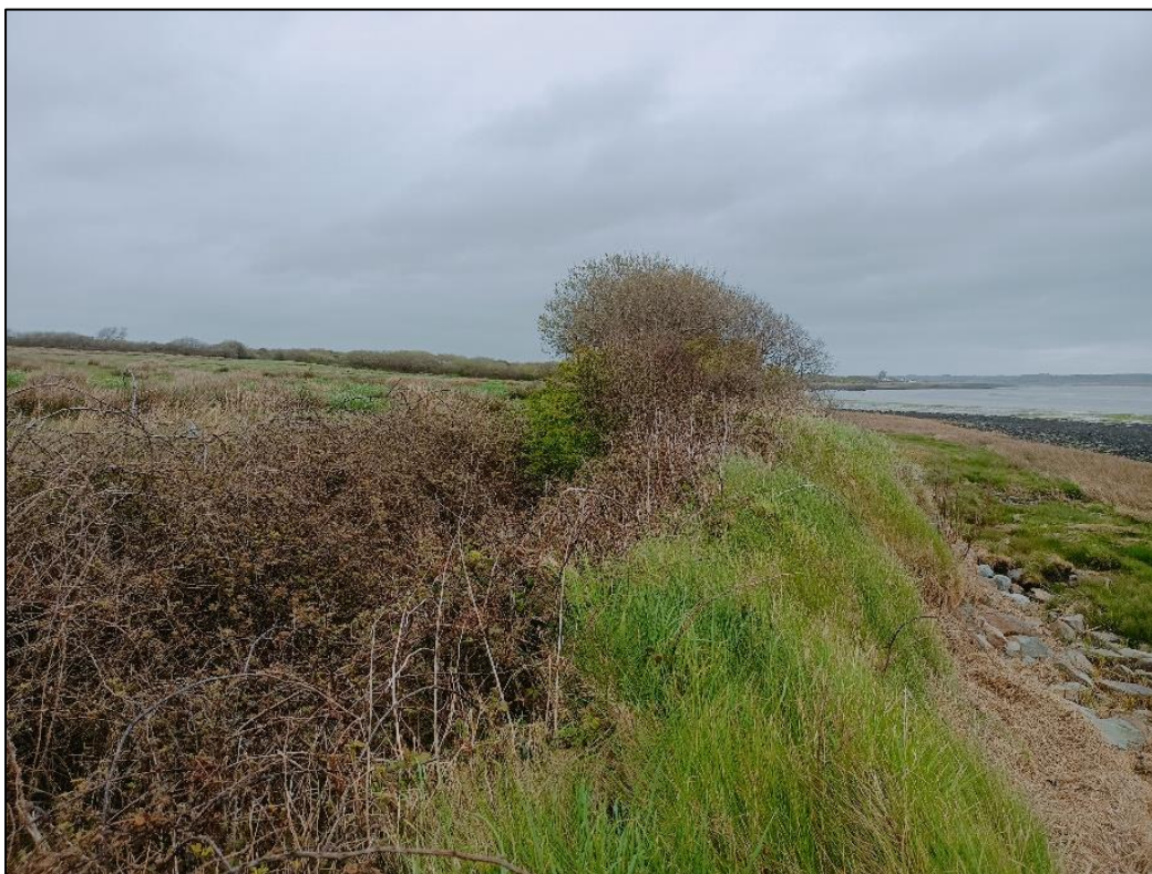
Plate 1.2 Ch. 5+420 looking east. Photo taken from bank.
