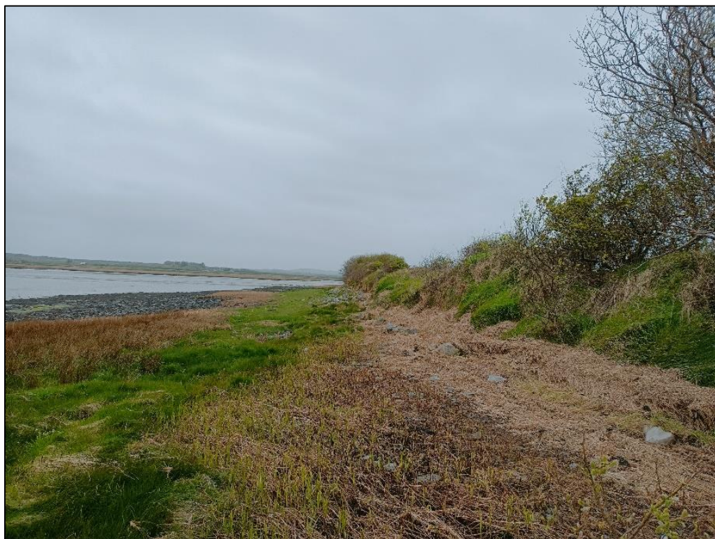
Plate 1.4 Looking west along shore at Ch. 5+550
