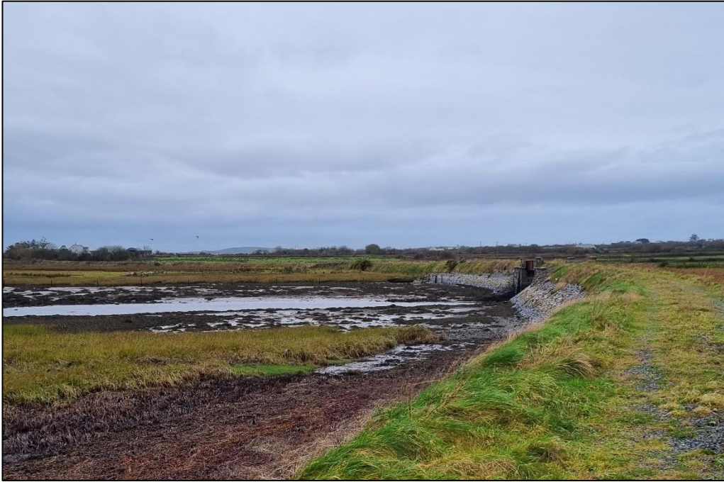
Plate 4.1. View west from east side of Moyasta Bridge
